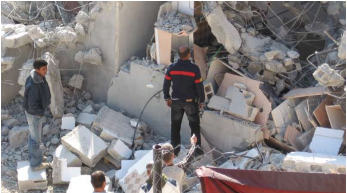
A Palestinian family looks through the remains of their demolished home in At Tur neighborhood. Photo by Gottfried Kraatz (EAPPI). December 2006.
