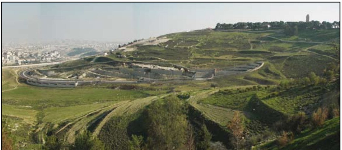
Mount Scopus Tunnel Road. 2007.
