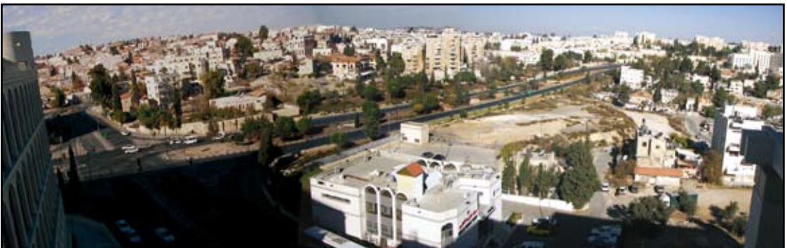
Municipal Road No. 1. 2007
